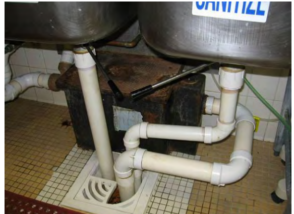
Photo #22: Cooking grease trap in Building 39
