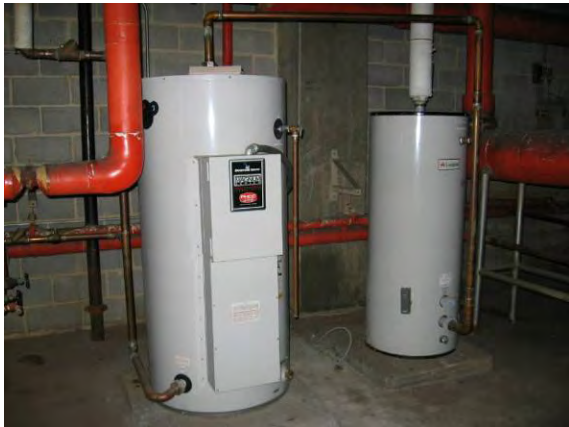
Photo #9: Electric domestic hot water heaters in each building
