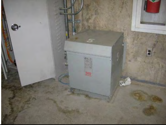
Photo #25: Step down transformer
