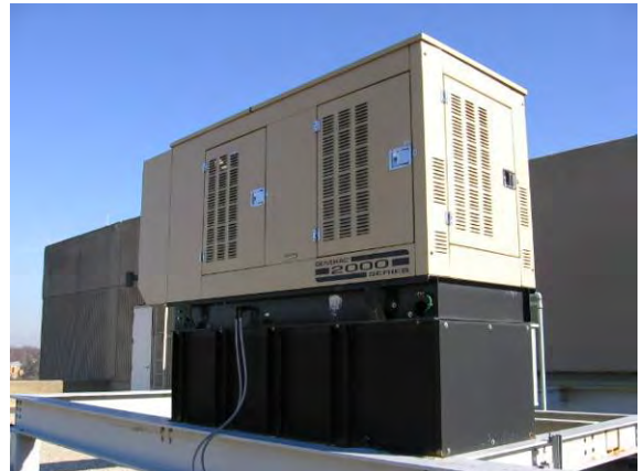
Photo #28: Homeland Security rooftop diesel belly tank for emergency generator on Building 41
