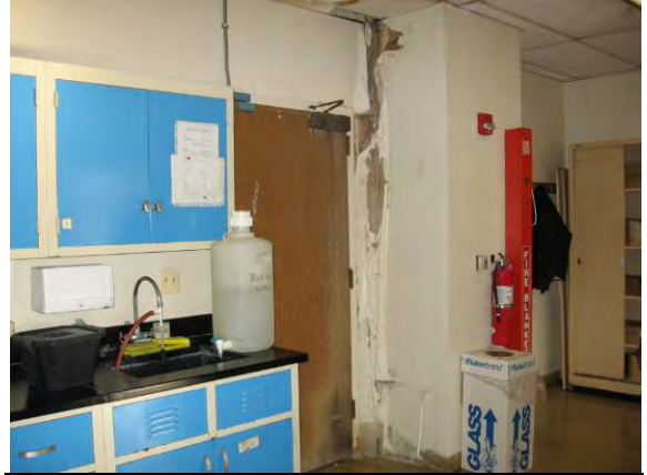
Photo #38: Water damaged ceiling tiles, drywall, and floor tiles in Building 44 Room 311
