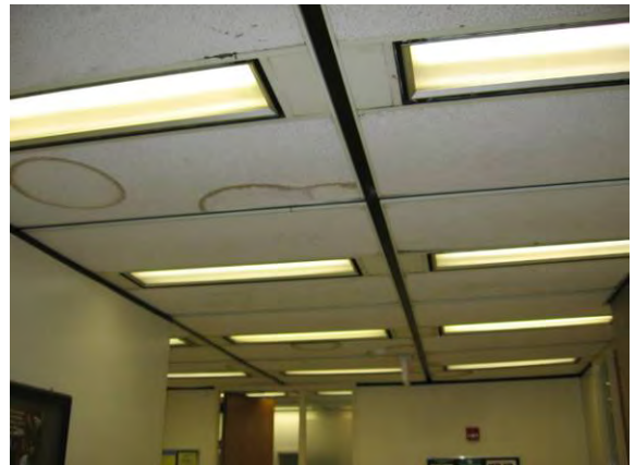
Photo #36: Water damaged ceiling tile in Buildings 38 and 39
