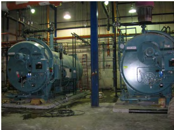
Photo #11: New natural gas and heating oil boilers in Building 43
