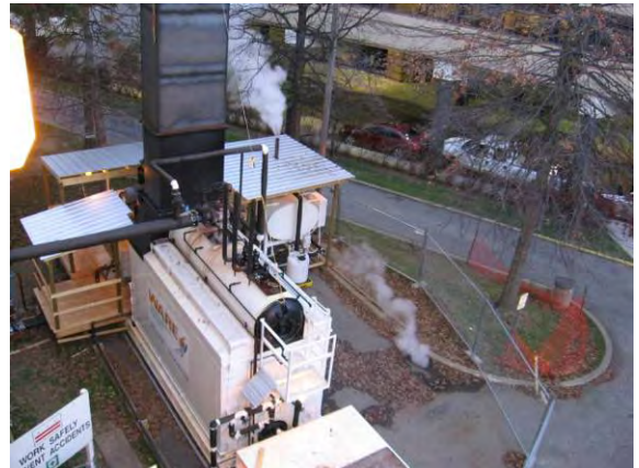
Photo #10: Temporary natural gas boiler at Building 43
