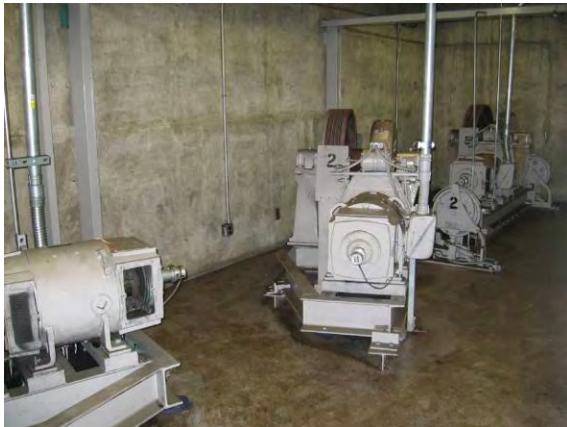
Photo #27: Two of 14 traction elevators at the Project
