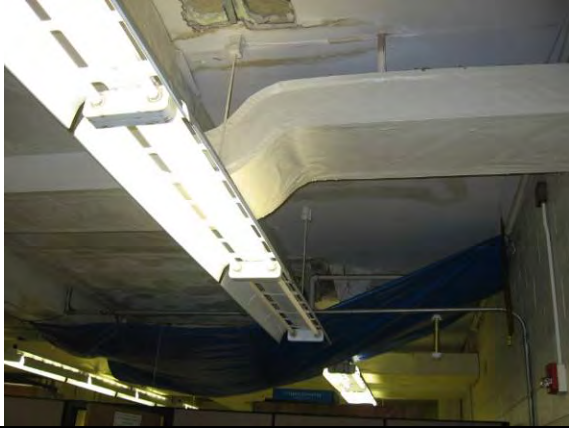
Photo #37: Water damaged painted drywall ceiling in the Building 39 copy room
