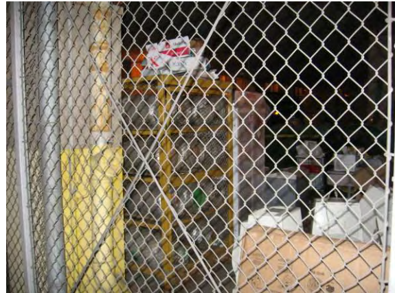
Photo #14: Propane cage for forklifts on the exterior of Building 42
