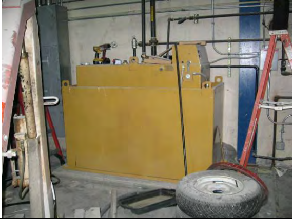
Photo #31: Emergency generator and 250-gallon day tank in Building 43
