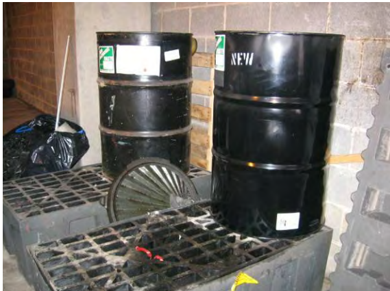
Photo #21: Waste oil 55-gallon drums with secondary containment at Building 43
