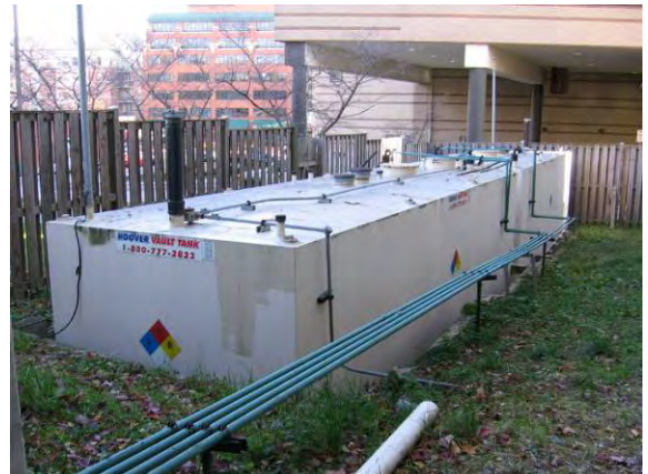
Photo #30: Two 8,000-gallon fuel oil ASTs (and former location of three 30,000-gallon USTs)
